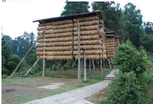
Figure 3: Preservation of Granaries Drying Racks
